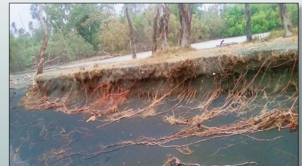
Increased Coastal Erosion due to Tropical Cyclone
